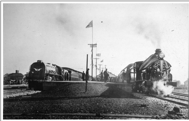
23.6.1937 - Port Pirie opening ( Commonwealth Railways )
