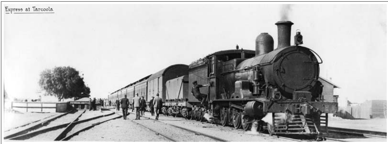
Tarcoola - Trans-Australian Railway G 2 on Trans-Australian (Chris Drymalik Collection)
