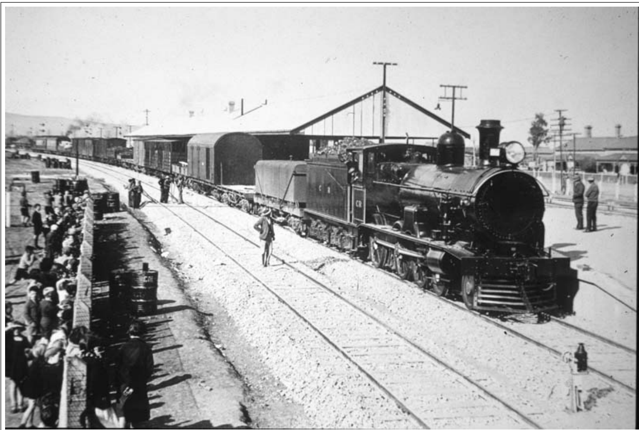
23.6.1937 - Port Pirie opening ( Commonwealth Railways )
