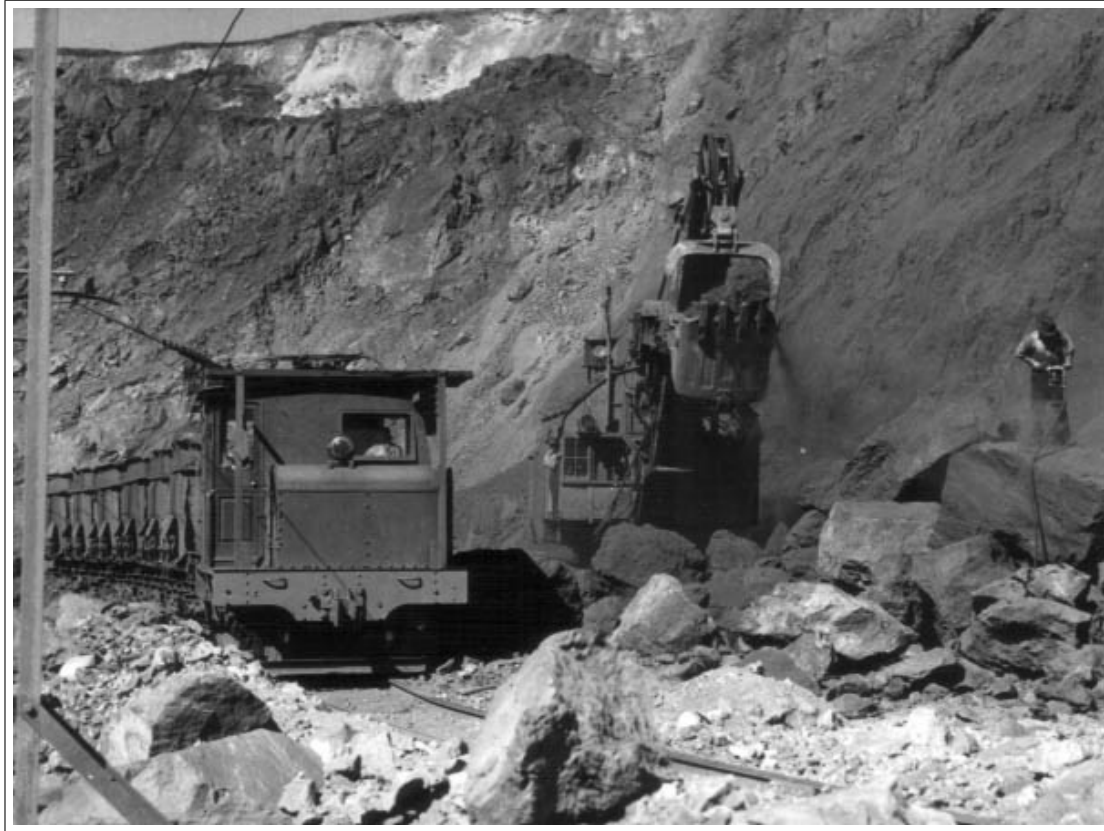
Broken Hill Proprietary Co. - Iron Knob Tramway - Electric Locomotive No. E1 - Metro-Vickers built, BHP electric loco No. 1 goes about its business at the Iron Knob quarry c.1930 ( NRM Collection )
