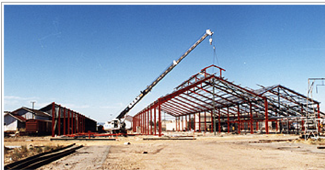
The current museum under construction ( NRM Collection )
