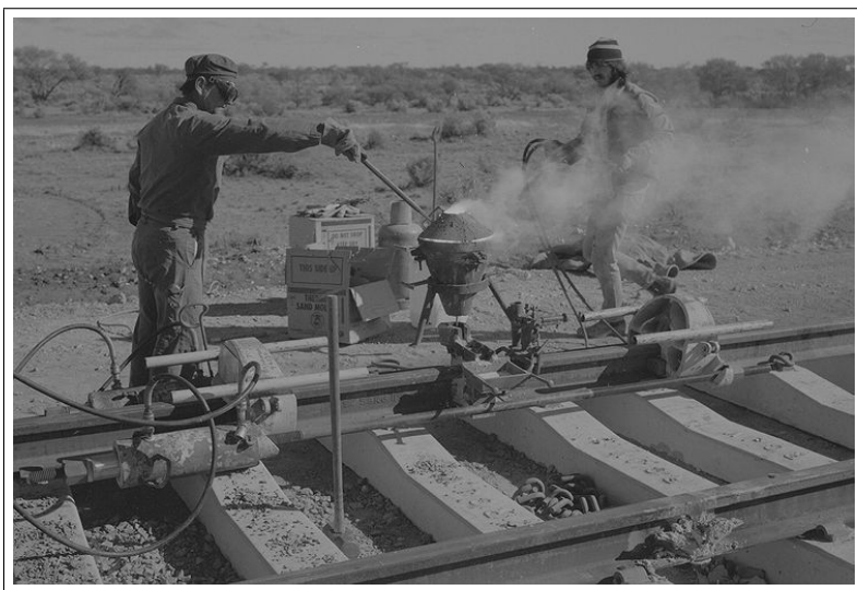
Building the Tarcoola to Alice Springs line ( NRM Collection )
