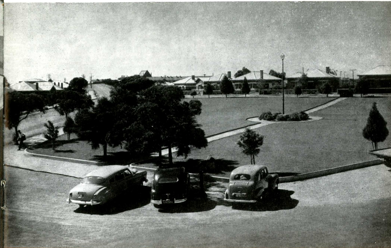
Commonwealth Railways Residences at Port Augusta.
