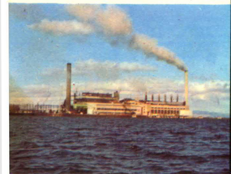
Thomas Playford Power Station, Port Augusta
